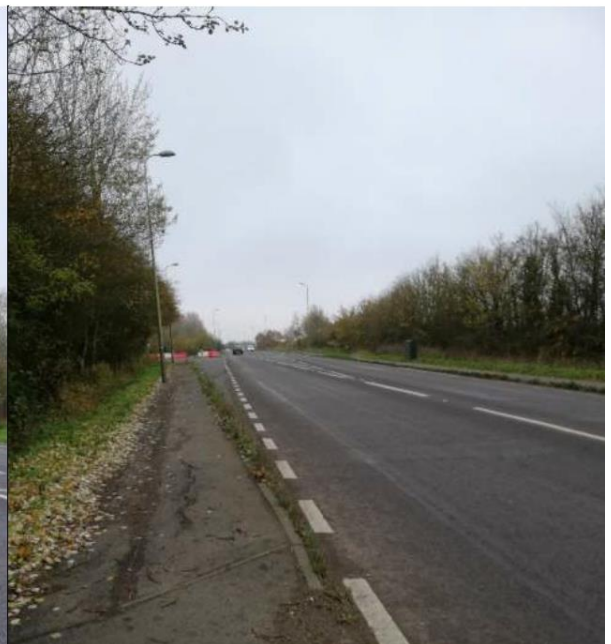
Photograph 2: A41 (East of Pioneer Road)
